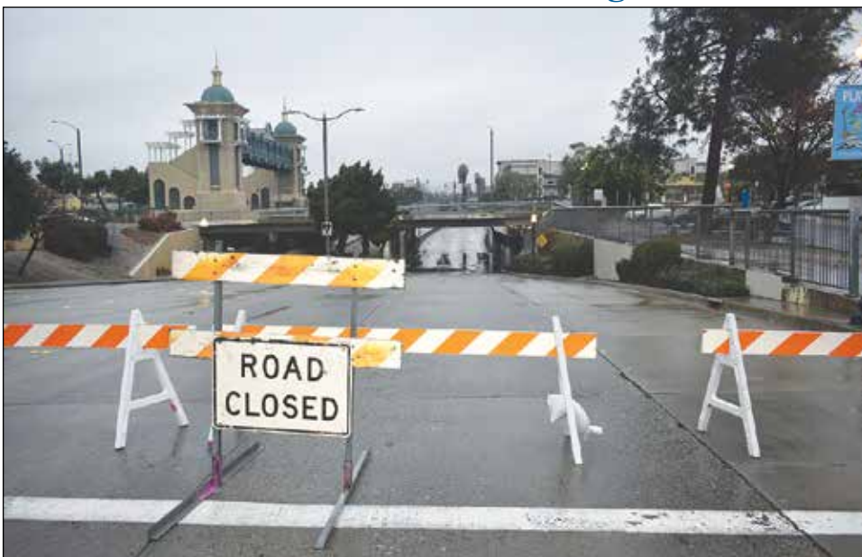
DOWNPOUR CLOSURES GAREY -- A Southern California Edison power line problem forced the early-morning closing of Garey Avenue between Second Street and Monterey Avenue during the rains this month. And later the same night, all of the undercrossings were closed -- Garey, Towne, Reservoir and East End -- as Pomona Public Works crews worked through the night to clear brush out of the drains.
