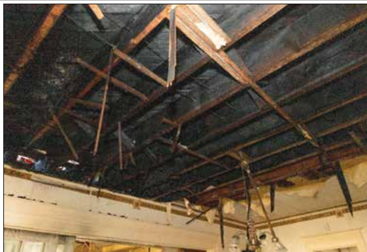
Interior damage from the fire is visible looking up toward the roof in the office area of the Ebell Museum building.
